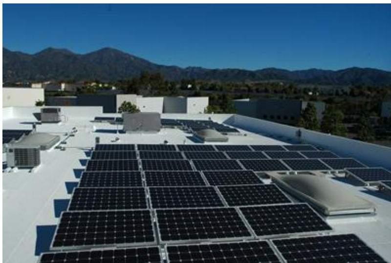
Roof with both reflective coating and solar Source: Cool Roofs Rating Council
