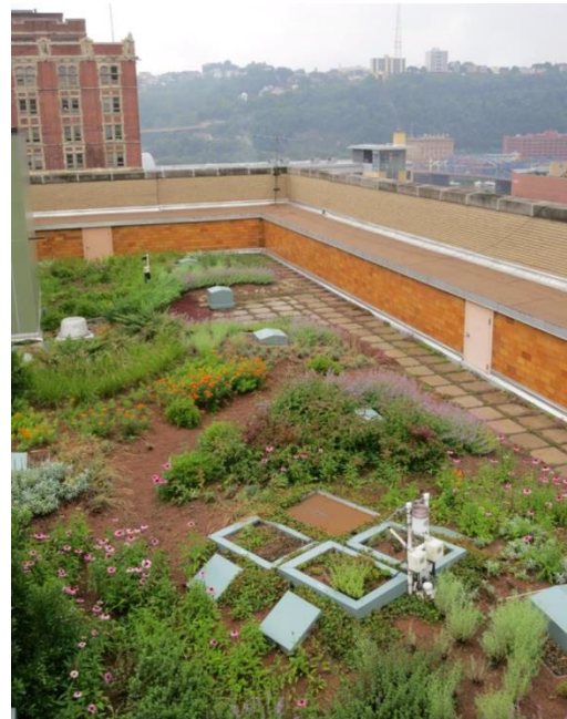
Green Roof on Allegheny County building
